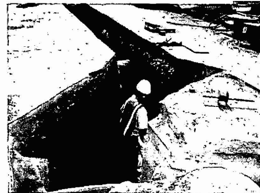
Workers install new natural gas pipeline in Jefferson City.
