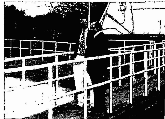
Jim Merciel and United Water Missouri manager John Hollenbach discuss plant operations.
